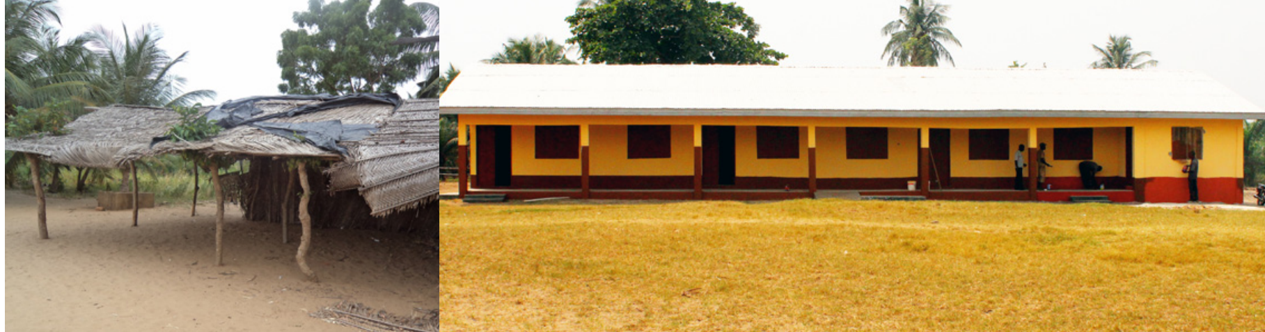
BEFORE, Avata Primary School
